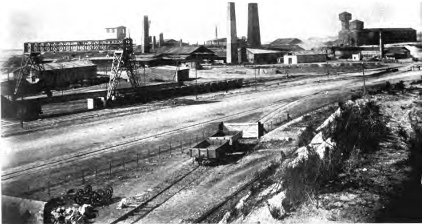
VIEW OF SMELTING WORKS, WALLAROO, LOOKING EAST.
